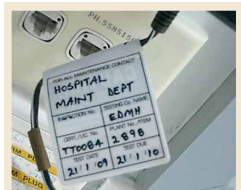
All electrical equipment in the hospital is tested and tagged to indicate that it is safe to use as part of the risk management strategy.
